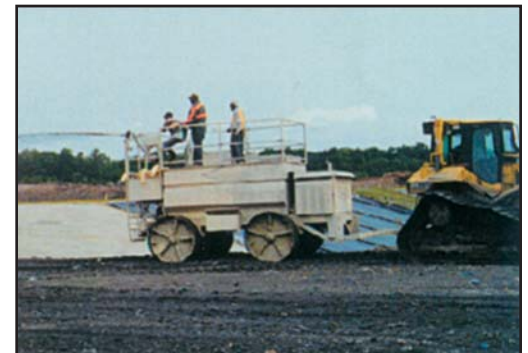
Solid waste received at the landfill is spread, compacted and covered with a spray foam (above) alternative daily cover or a six-inch layer of soil at the end of each work day.
